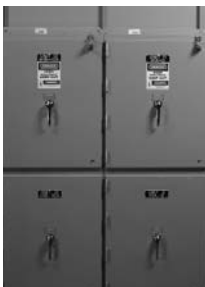
The arc resistant rear doors and plenum of a two-high design.
